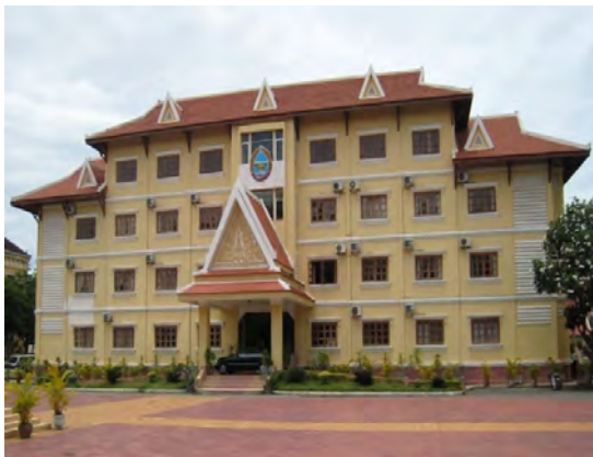
Battambang Provincial Hall
